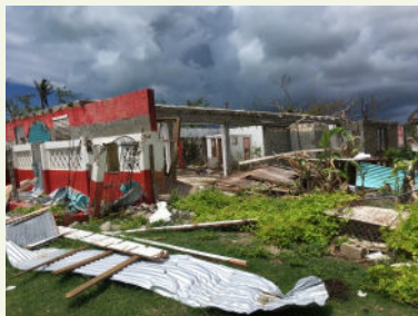
Hurricane Irma Damage in Barbuda
