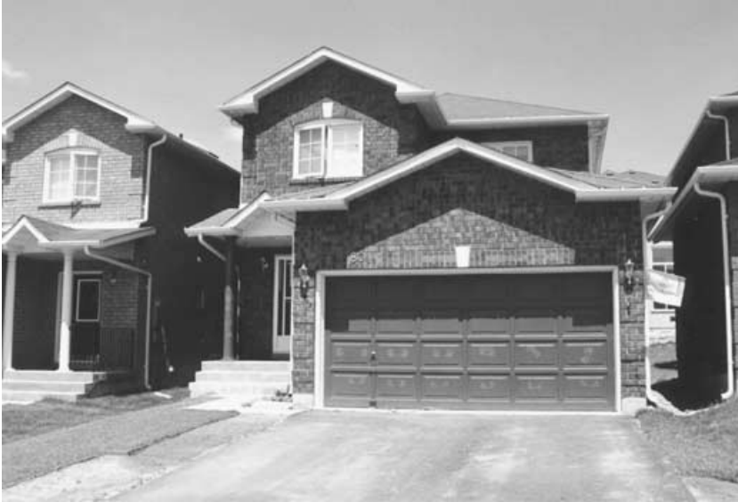
FIG. 1. A typical single-family home in Netville.
